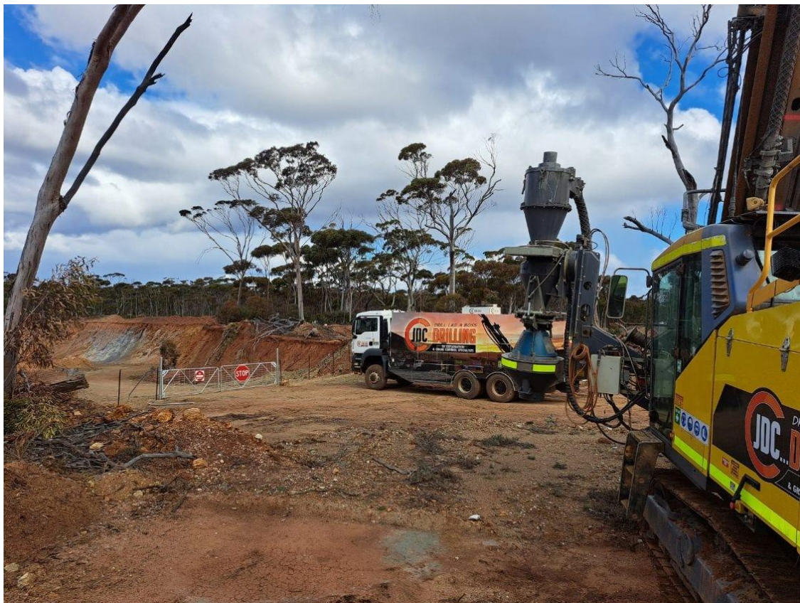
Figure 1 – Drill Rig arrives onsite at Van Uden
