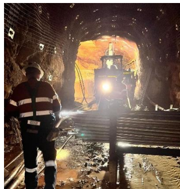
Figure 1: Underground ground support preparations
