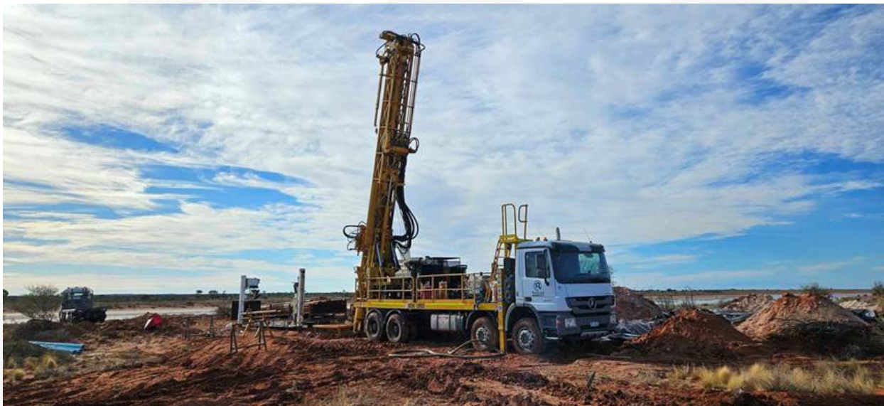
Plate 1 – Diamond drill rig set up on 25FNDD011
