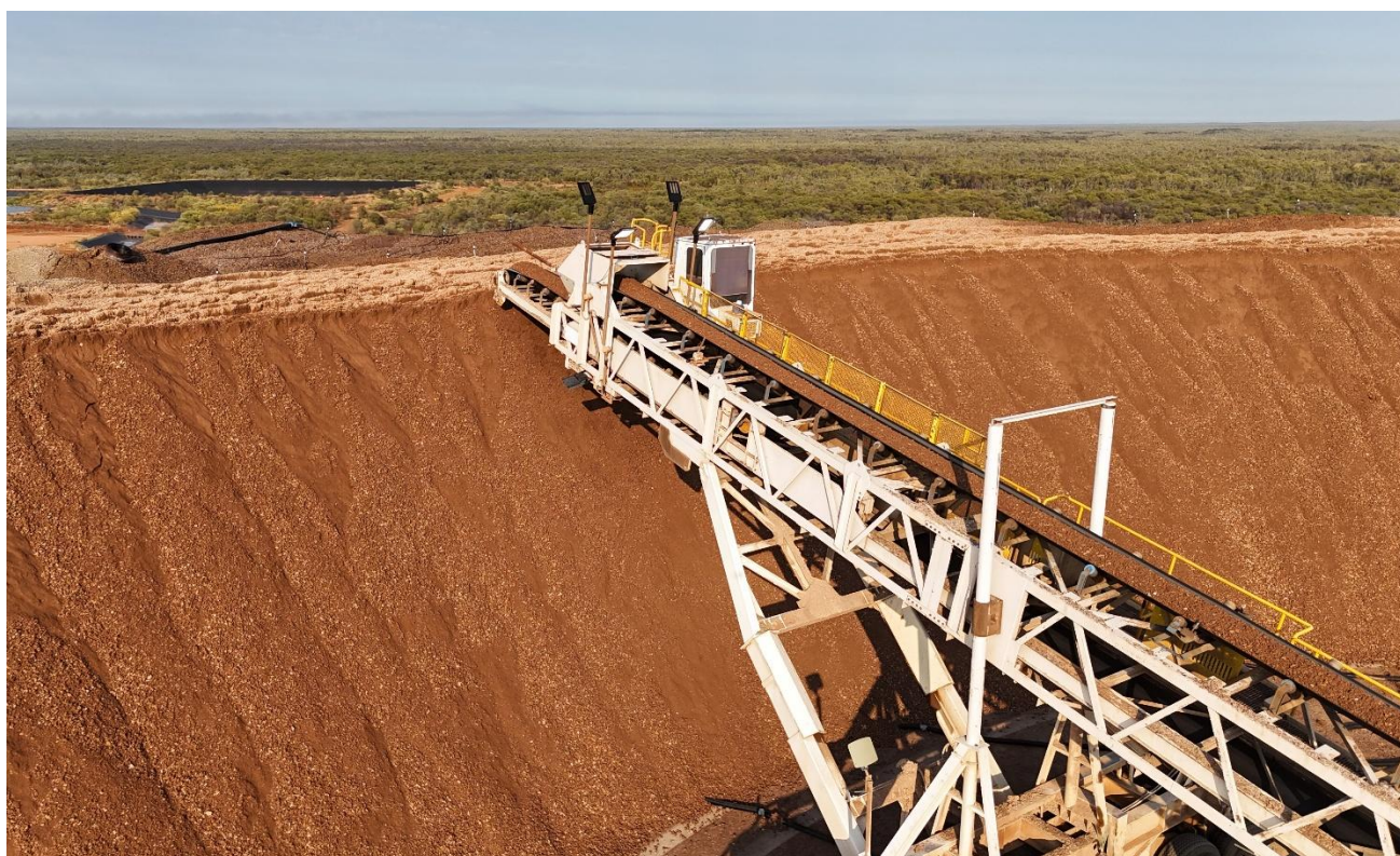
Figure 3: Heap Leach Pad 18 Stacking
