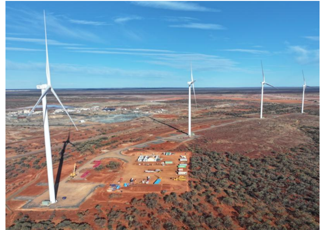
Windfarm – turbine installation commissioned
