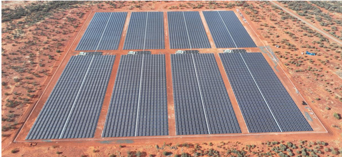
Solar – 27MW solar installation commissioned
