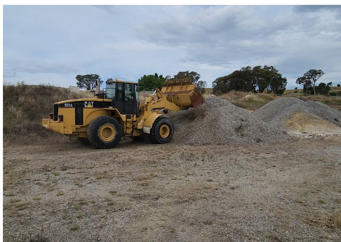
Above: Loader after being repaired on site.
