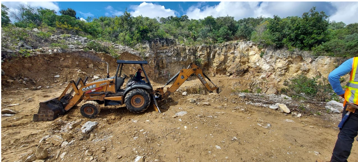
Clean up pits for fresh rock exposure
