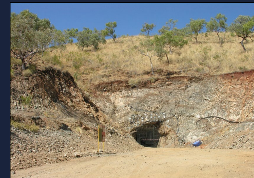
Panton mining portal
