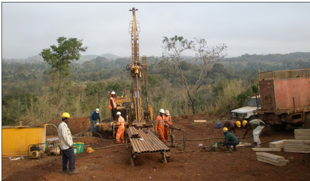
Figure 22: Diamond drilling at Firawa
