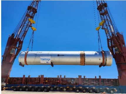
Acid Bake Kiln (weight 100 tonnes)
