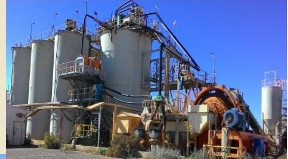
Processing Plant & Infrastructure in Laverton
