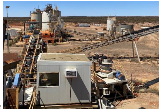
Laverton Processing Plant. May 2023
