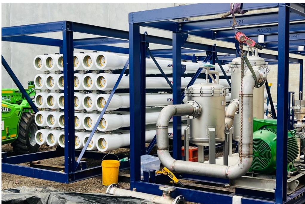
Figure 1. Construction of Nano-filtration Plant in Sydney is well advanced.
