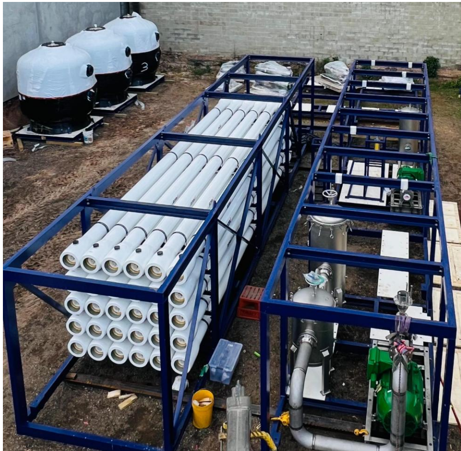
Figure 4. Assembly of Nano-filtration plant and filters in Sydney.
