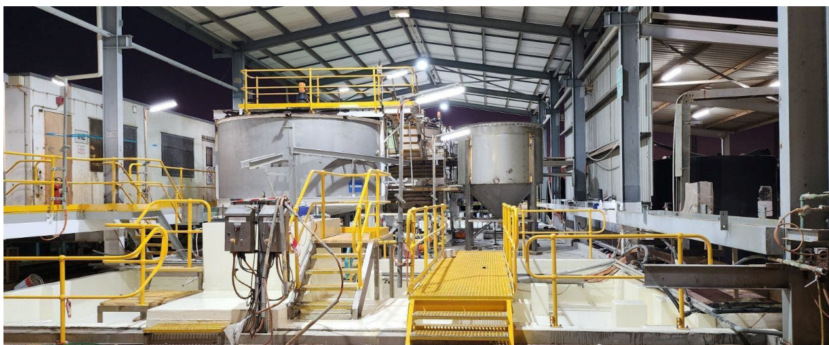
Figure 1. Solvent Extraction Crystal Plant post refurbishment
