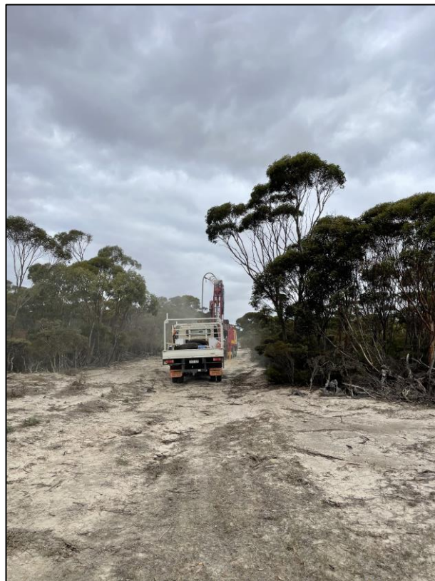
Figure 2 & 3: Drilling Activities at Pink Bark
