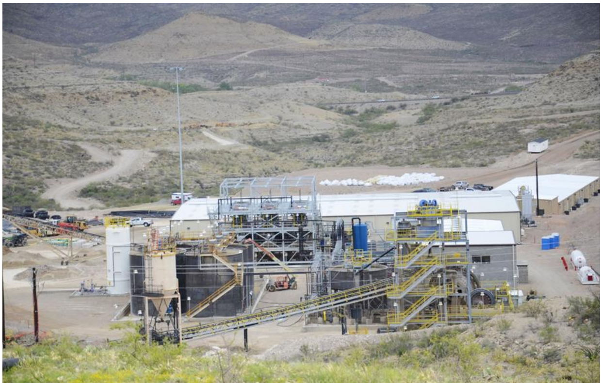
Figure 5: Shafter Processing Infrastructure.
