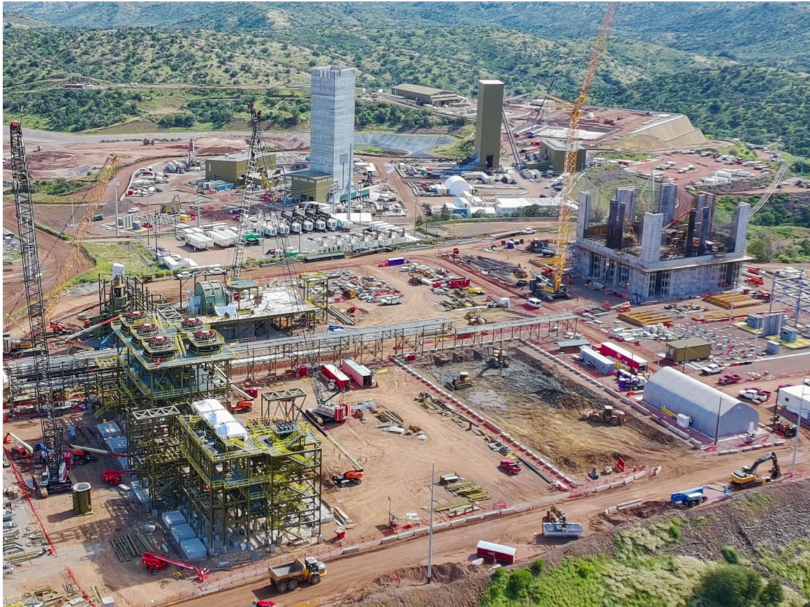
Taylor process plant construction (looking north)
