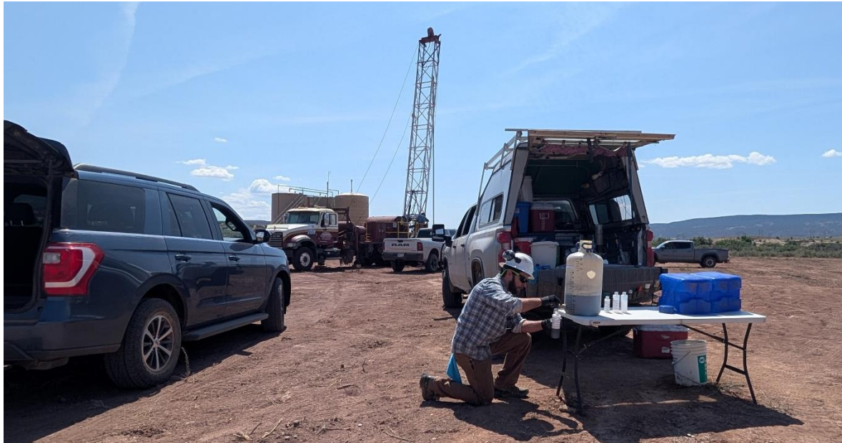
Figure 2: Evelyn Chambers #1 well – sampling and on-site testing
