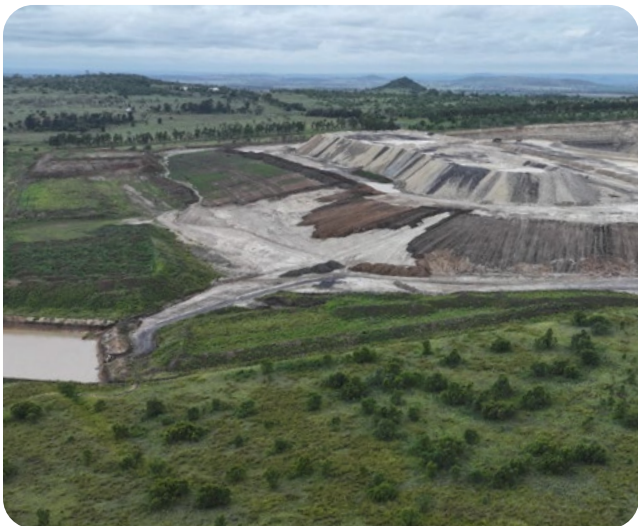
Rehabilitation at Willeroo Pit, New Acland, January 2026.
