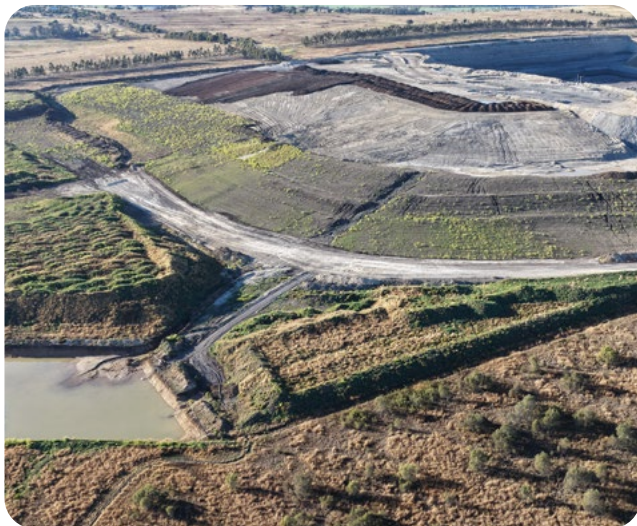
Rehabilitation at Willeroo Pit, New Acland, August 2026.
