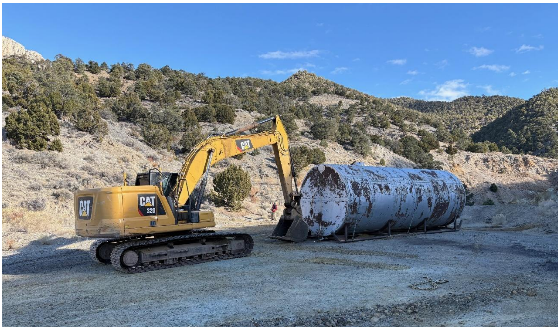
Water tank being positioned for drilling programme
