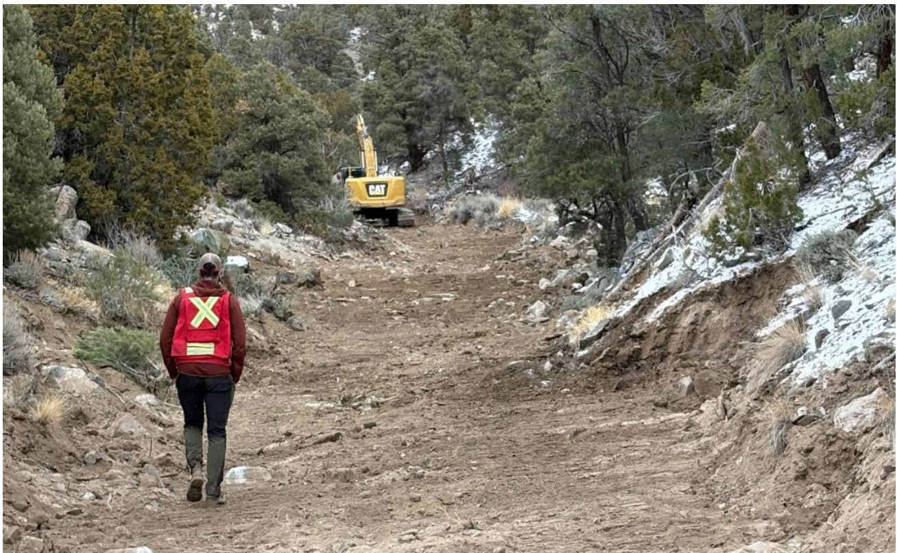
Figure 1: Wasp target drill site access earthworks.
