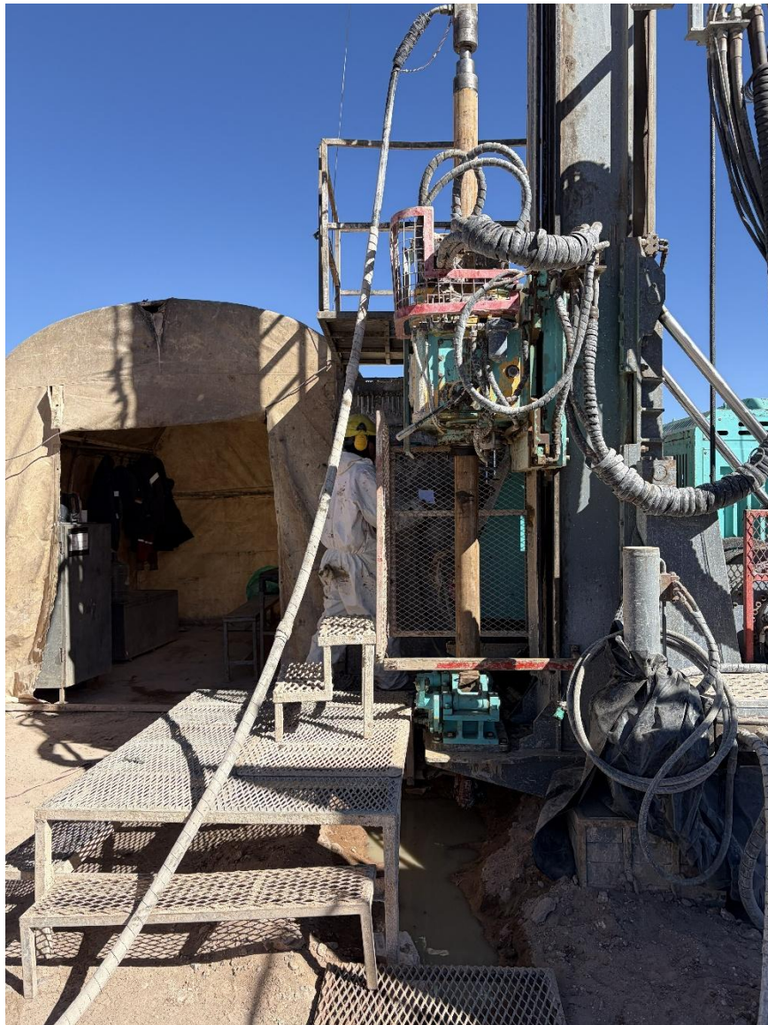
Figure 1. Well 9 being drilled with PQ diameter diamond drill before being reamed with 6 1/2inch tricone bit.
