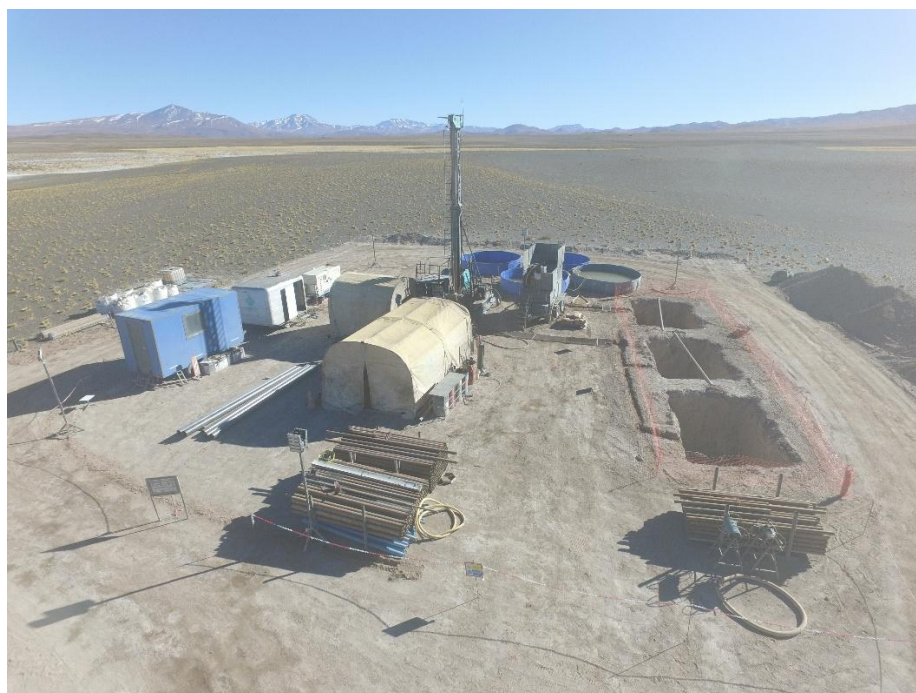
Figure 3. Drill site with sump ponds dug and pipe delivered. We don't need a camp as we are 10km from Jama town.
