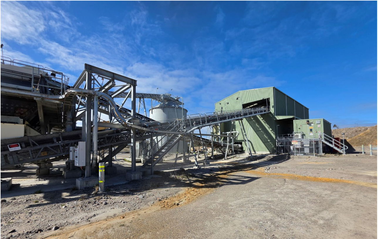
Figure 4: View from the triple-deck screen looking back towards the primary crushing and materials handling infrastructure
