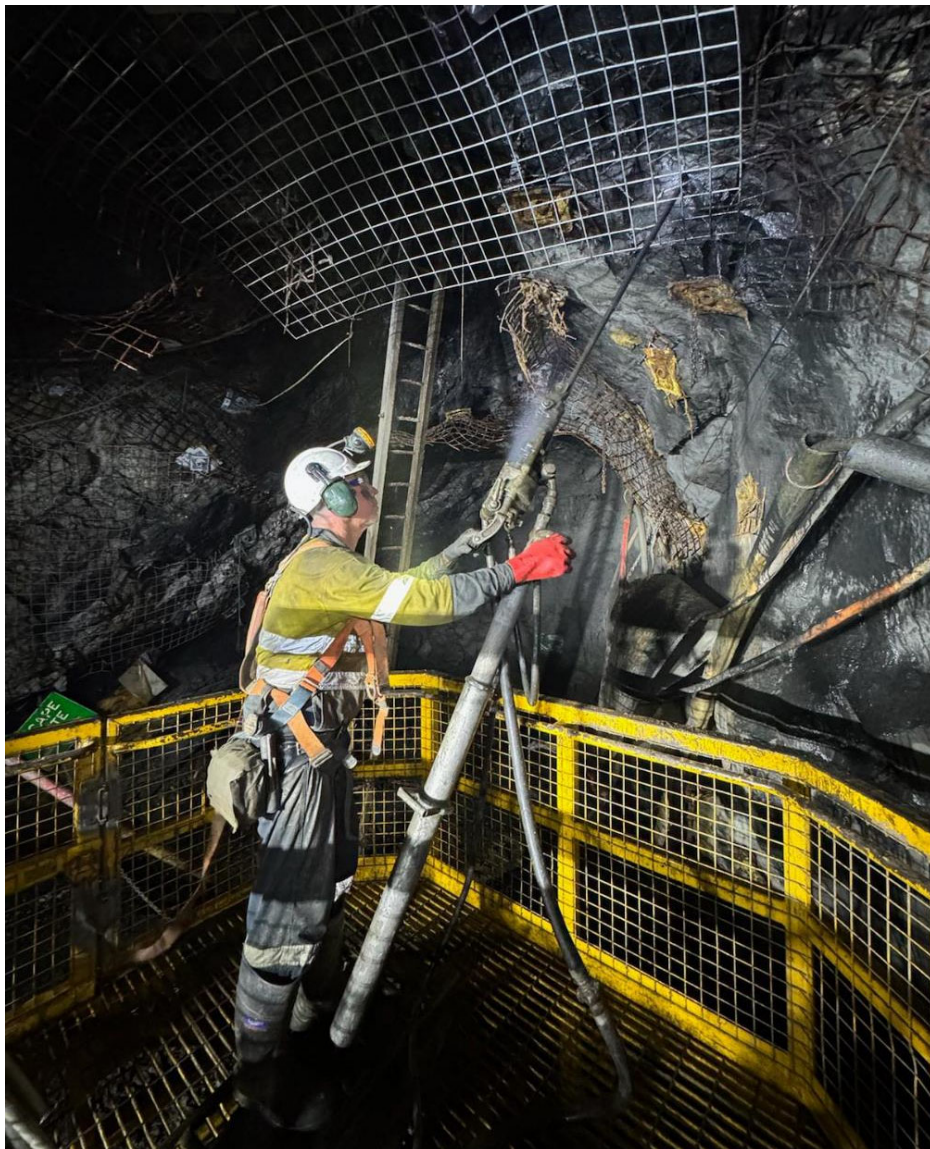
Figure 4: Cream Mining's Michael Duffy completing escapeway rehabilitation works at Paulsens underground
