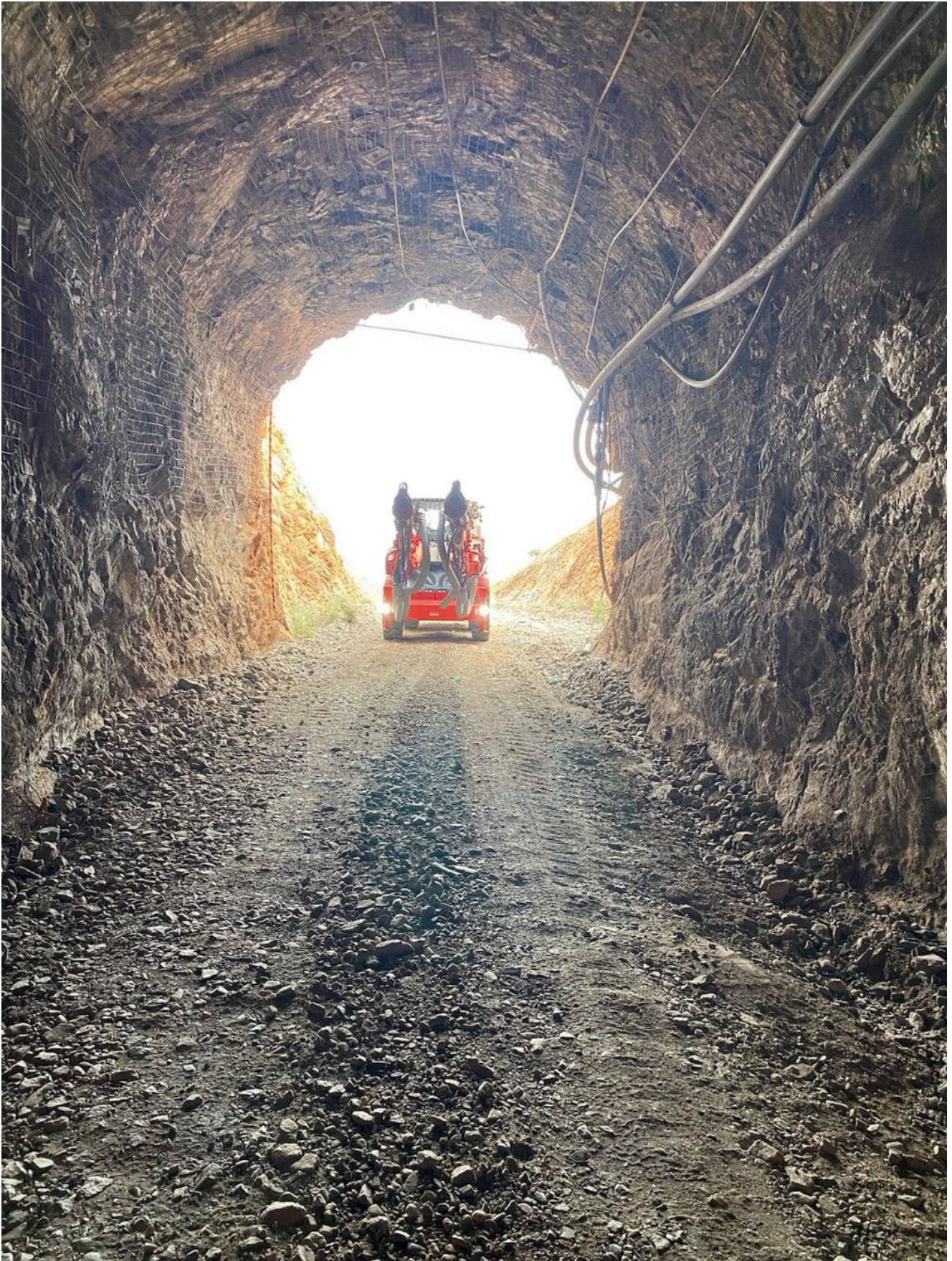
Figure 7 Twin boom jumbo mobilising into Paulsens underground portal for commissioning and rehabilitation activities
