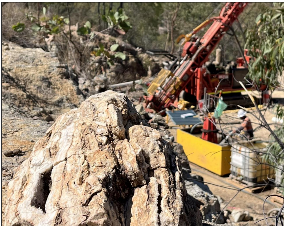
Figure 2: Hole 25FCDD001 collared at Francis Creek, Sybil.
