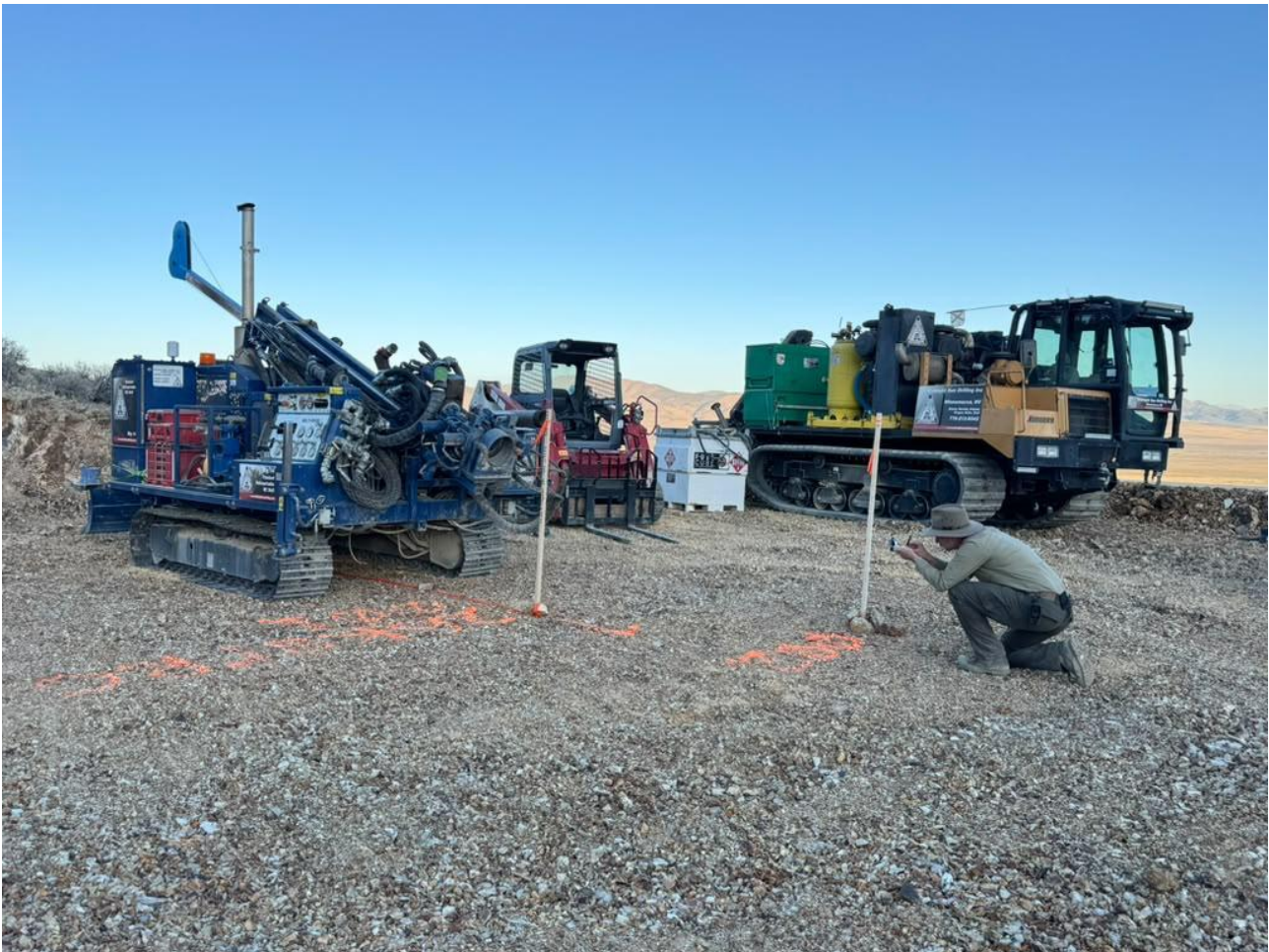
Figure 1: RC Drill rig successfully mobiles to the Keystone Project, Nevada
