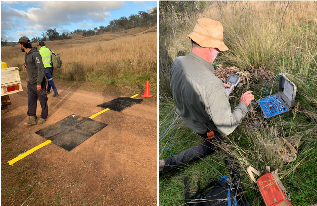
Figure 1 (L) and 2 (R) : Laying cabling, the main cable with road protection (L), geophysicist recording dipole readings (R)
