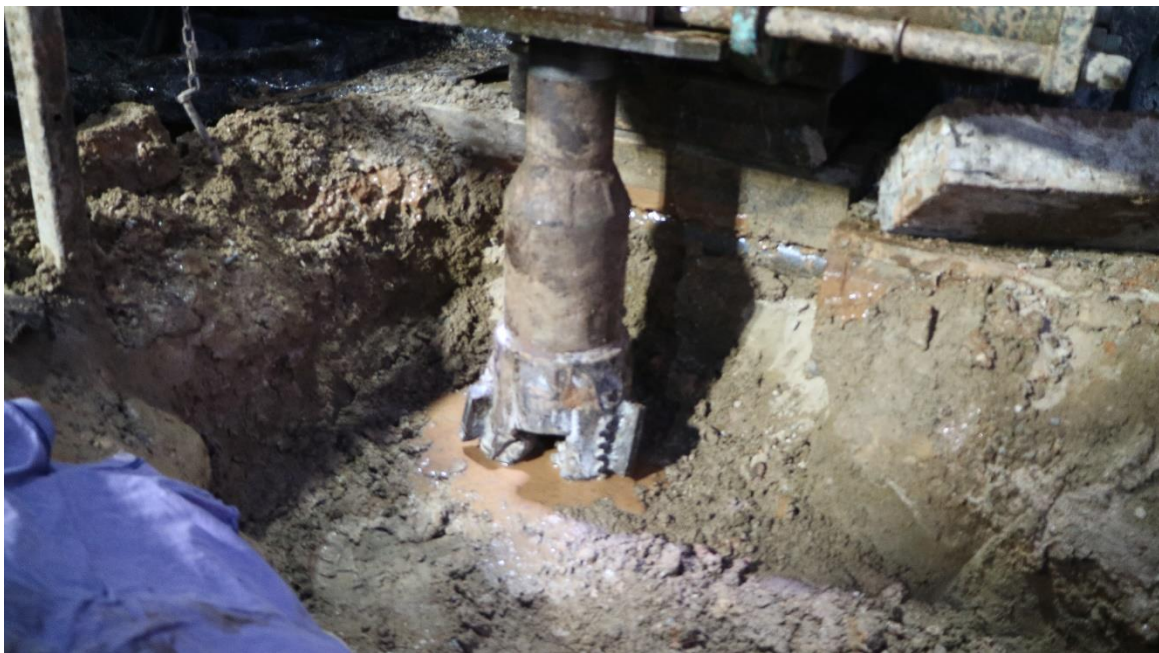
Figure 1. 9 3/4 tricone drill bit reaming out well for slotted pvc lining and filter material around pipe.
