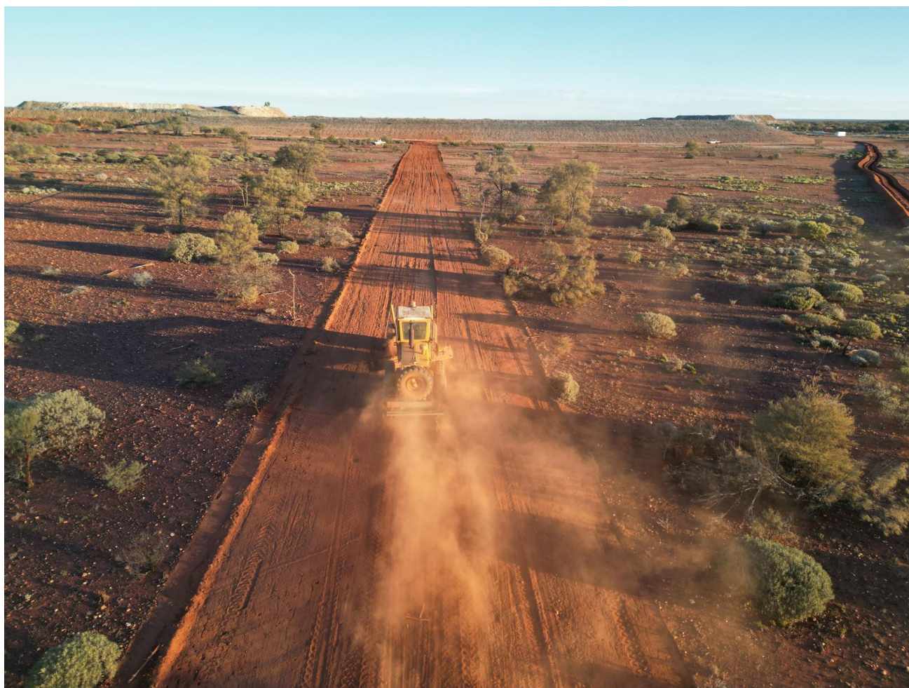
Figure 1: Haul road construction underway, July 2024.
