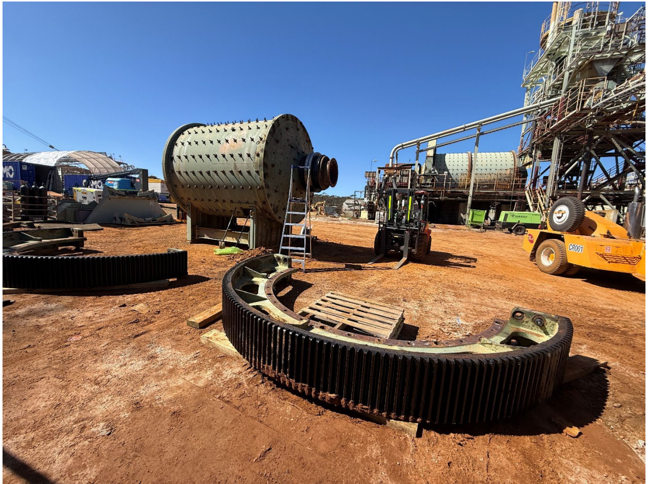
Image 2: Lake Johnston Mill Refurbishment
