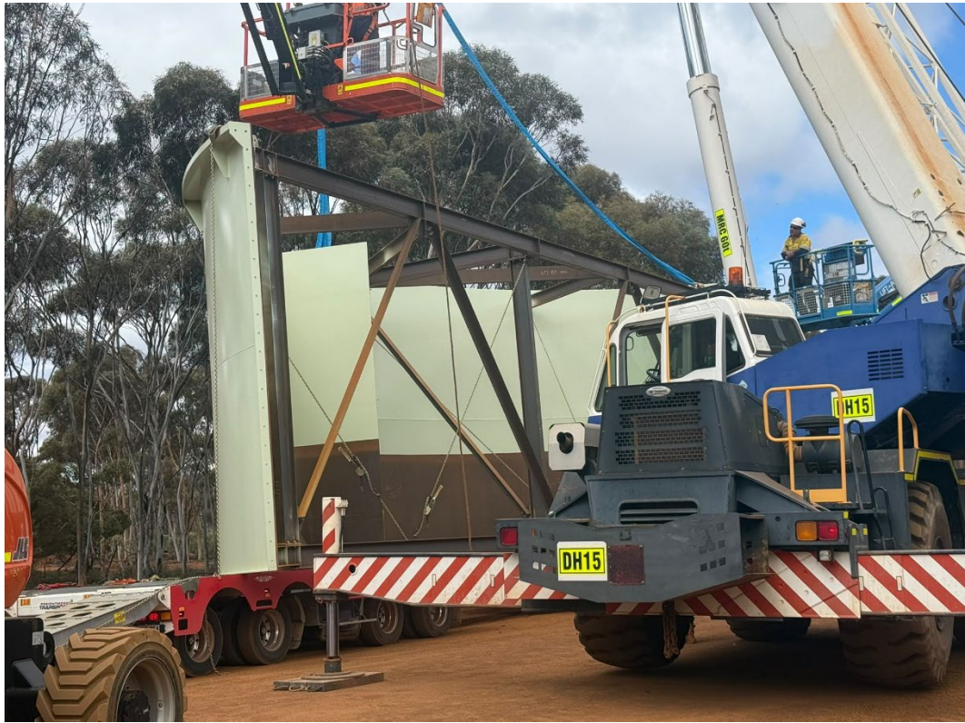
Image 4 & 5: Lake Johnston Processing Facility – CIL tank sections
