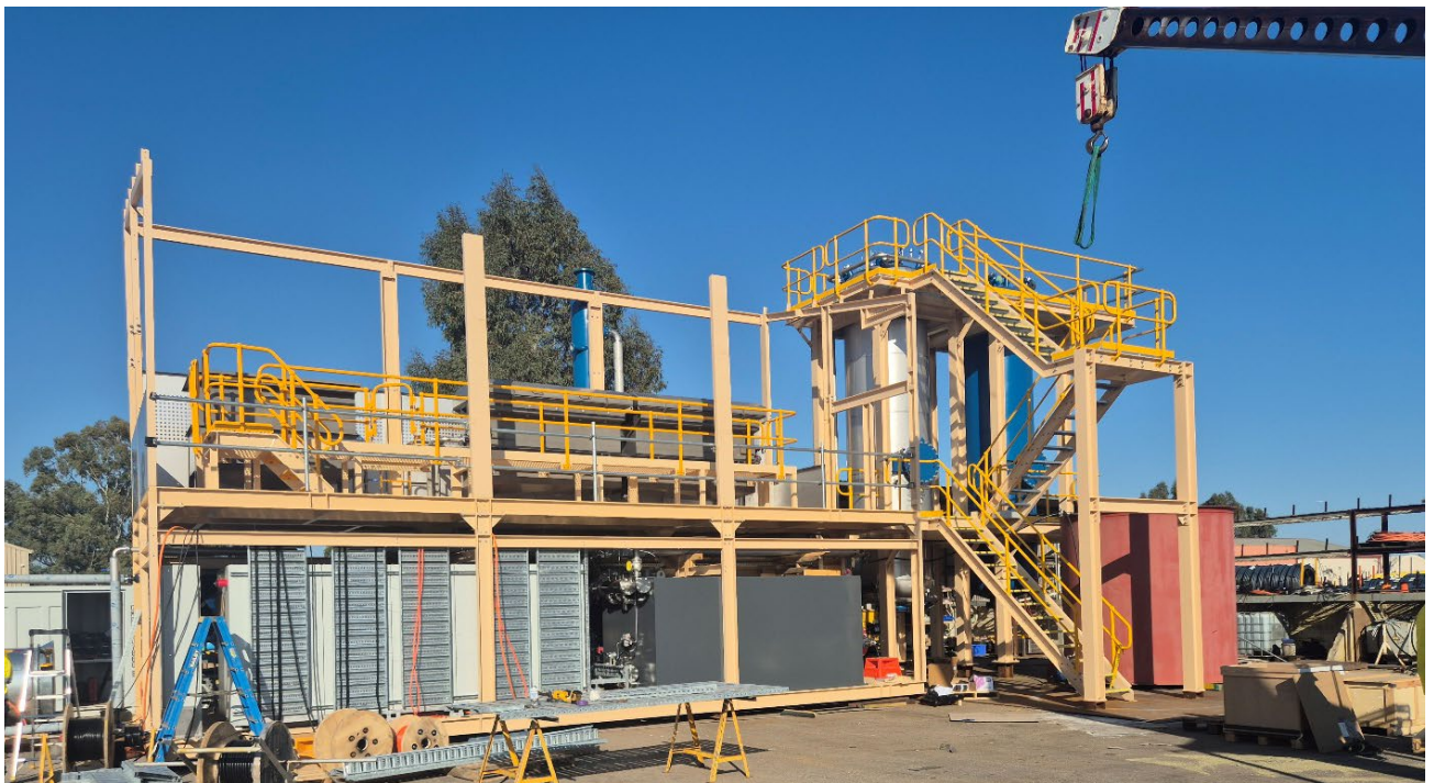
Image 3: Fabrication of Modularised Gold Elution Plant in Maddington, WA
