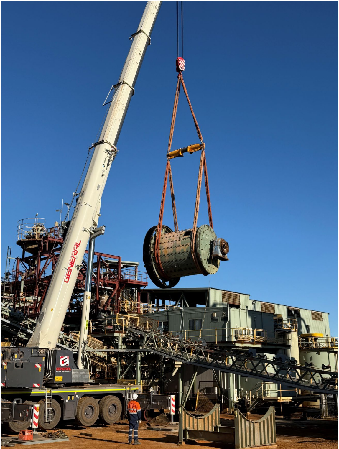
Image 1: Mill Refurbishment significantly advanced
