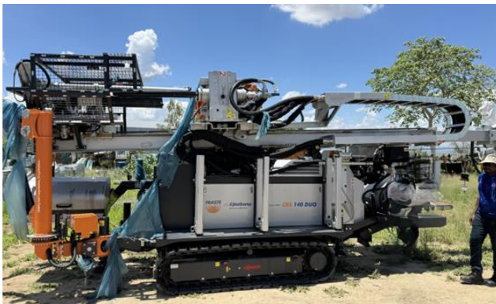
Figure 3- Sonic Rig 2 arrival at site
