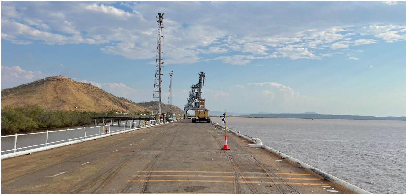
Figure 10: Wharf at Wyndham Port
