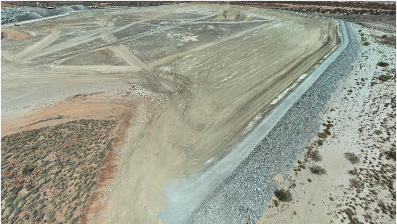
Figure 6: Showing the completed lift on the tailings storage facility facing East.
