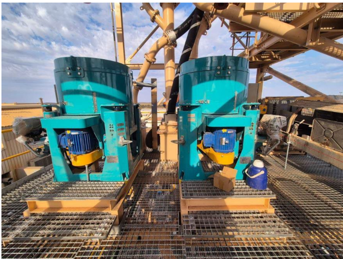
Figure 2: Showing the new, installed Knelson gravity concentrators.
