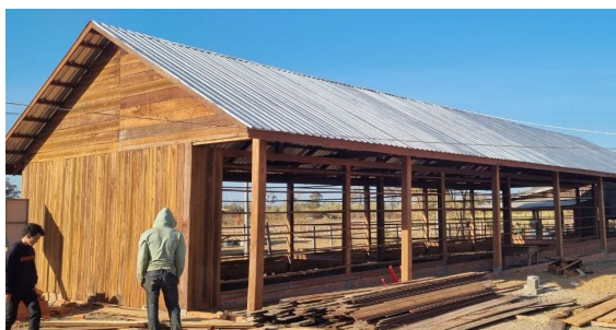
Figure 45 | New roof on school building
