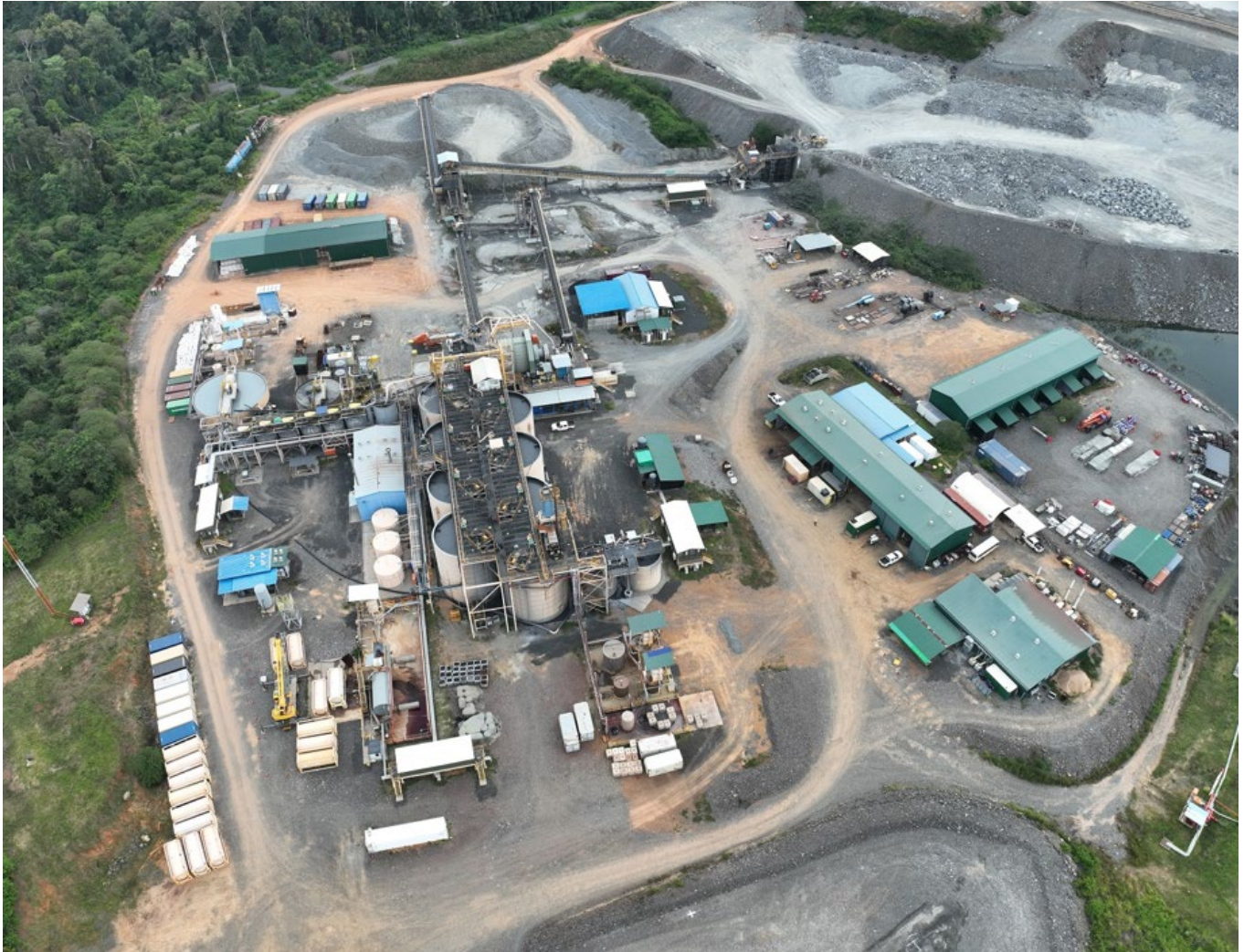
Figure 7 | Okvau Processing Plant
