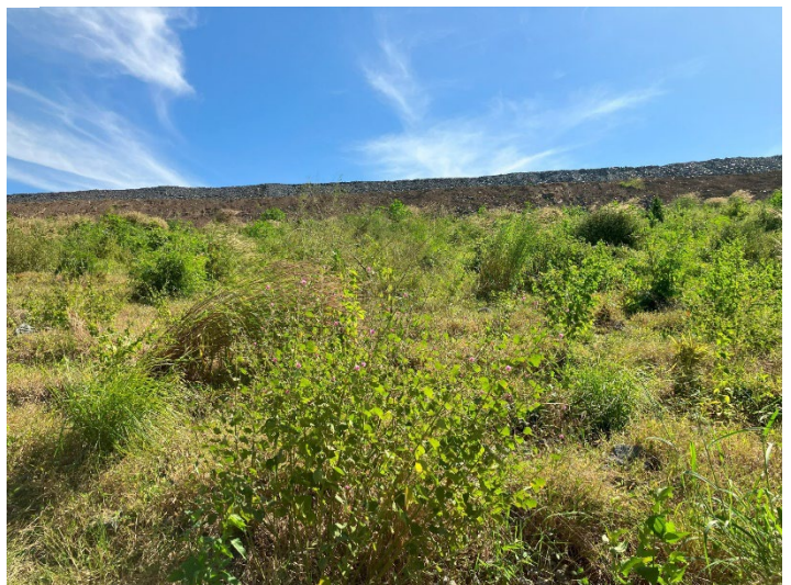
Figure 38 | Okvau waste rock dump under rehabilitation
