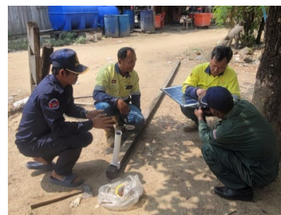
Figure 47 | Installing roadside lighting
