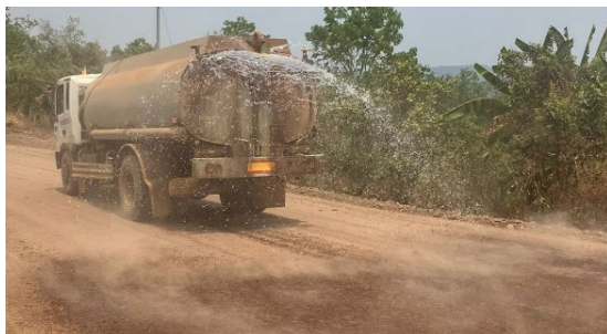
Figure 48 | Dust suppression on community road
