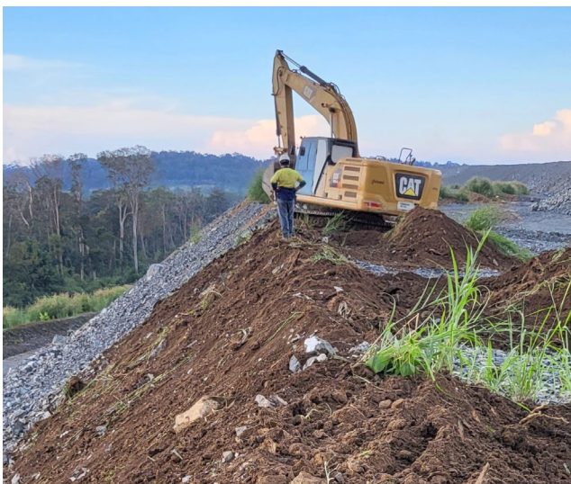
Figure 37 | Okvau batter/berm trial
