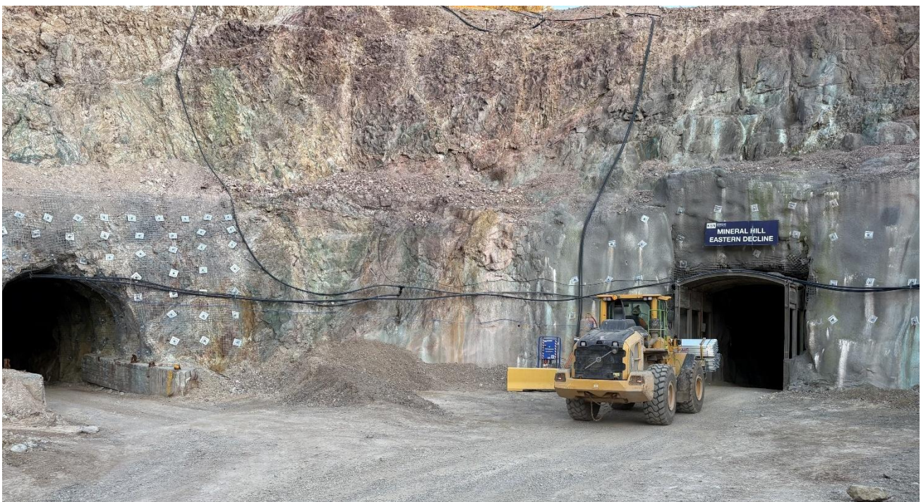
Figure 4: Jack's Hut Portal (Left) – originally mined in 1992. Rehabilitation of the portal and the initial 150m of decline are complete. EOZ (right) development rehabilitation is nearing completion, providing access to the initial production areas in the SOZ.
