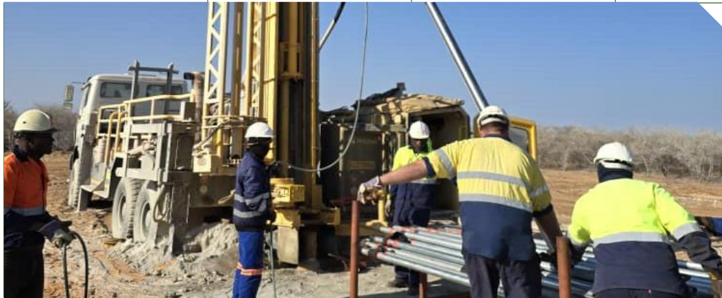
Injection well drilling, Ngami Copper Project
