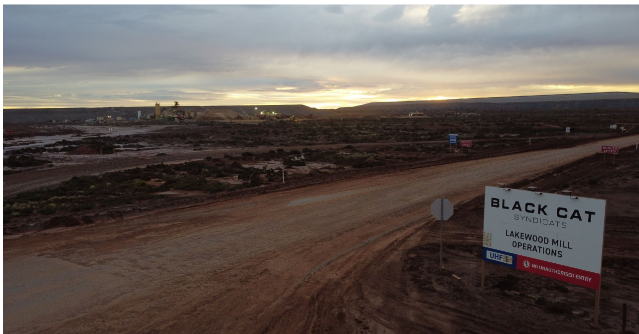
Figure 1: Lakewood processing facility
