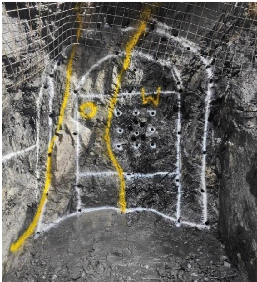
Photo 7. Montezuma exploration drive heading marked-up and ready to be charged
