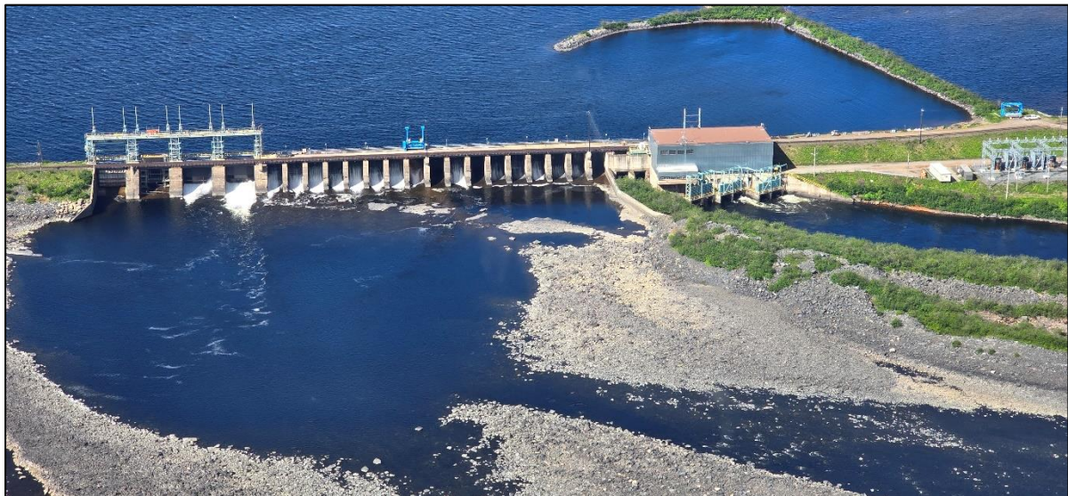
Figure 13: Menihek Hydropower Plant
