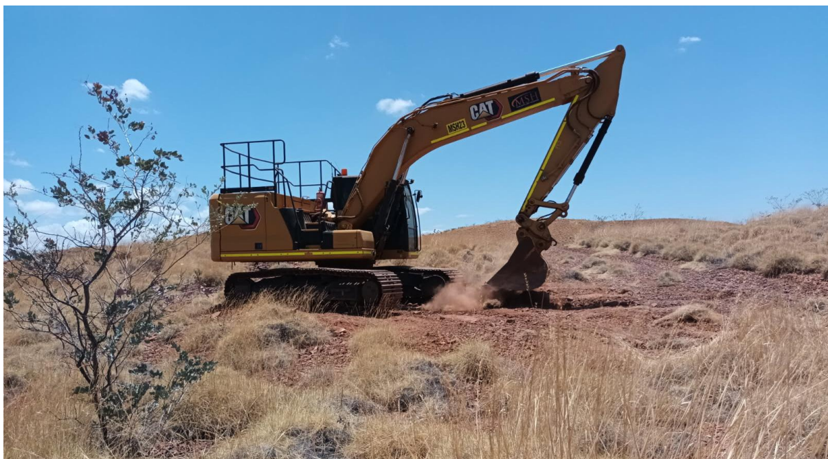
Photo 2: Establishing Drill Pad for Phase 1 Drill Program
