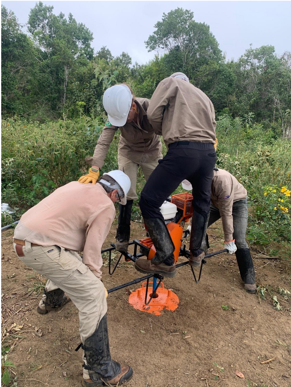
Figure 2. Drilling in progress on an auger hole at Irajuba Prospect
