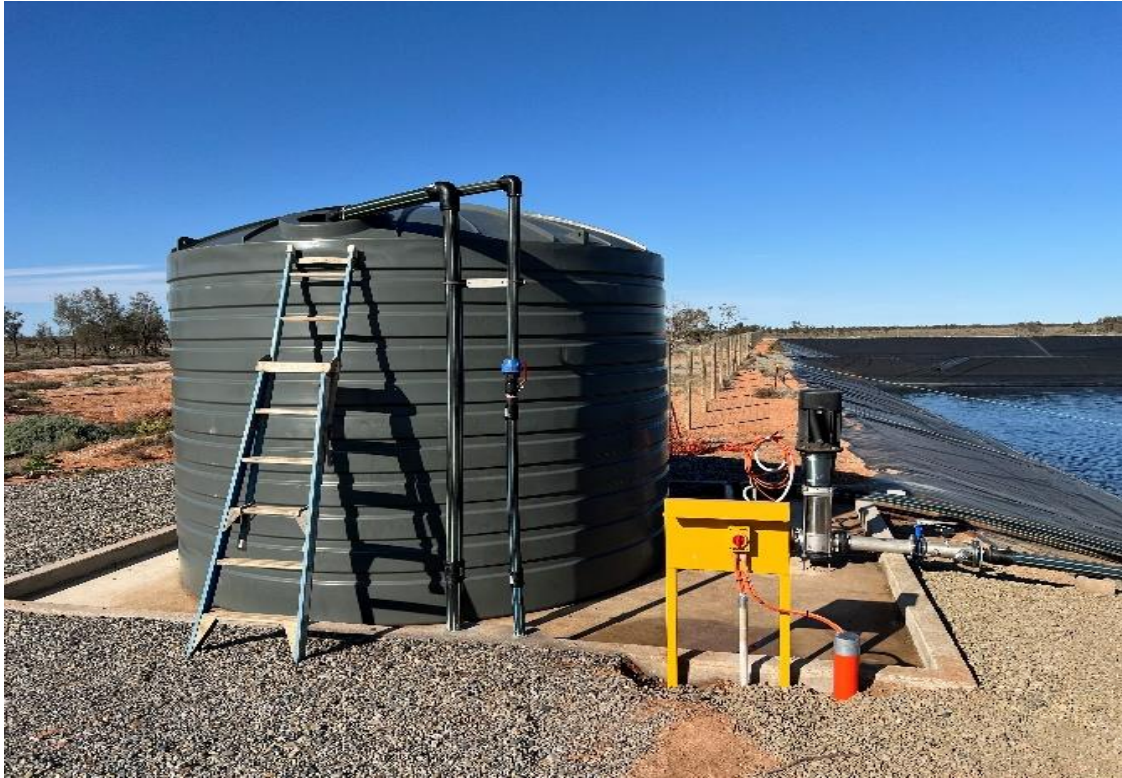
Figure 36: Installation of concrete bunds around raw water tanks as part of environmental management at White Dam
