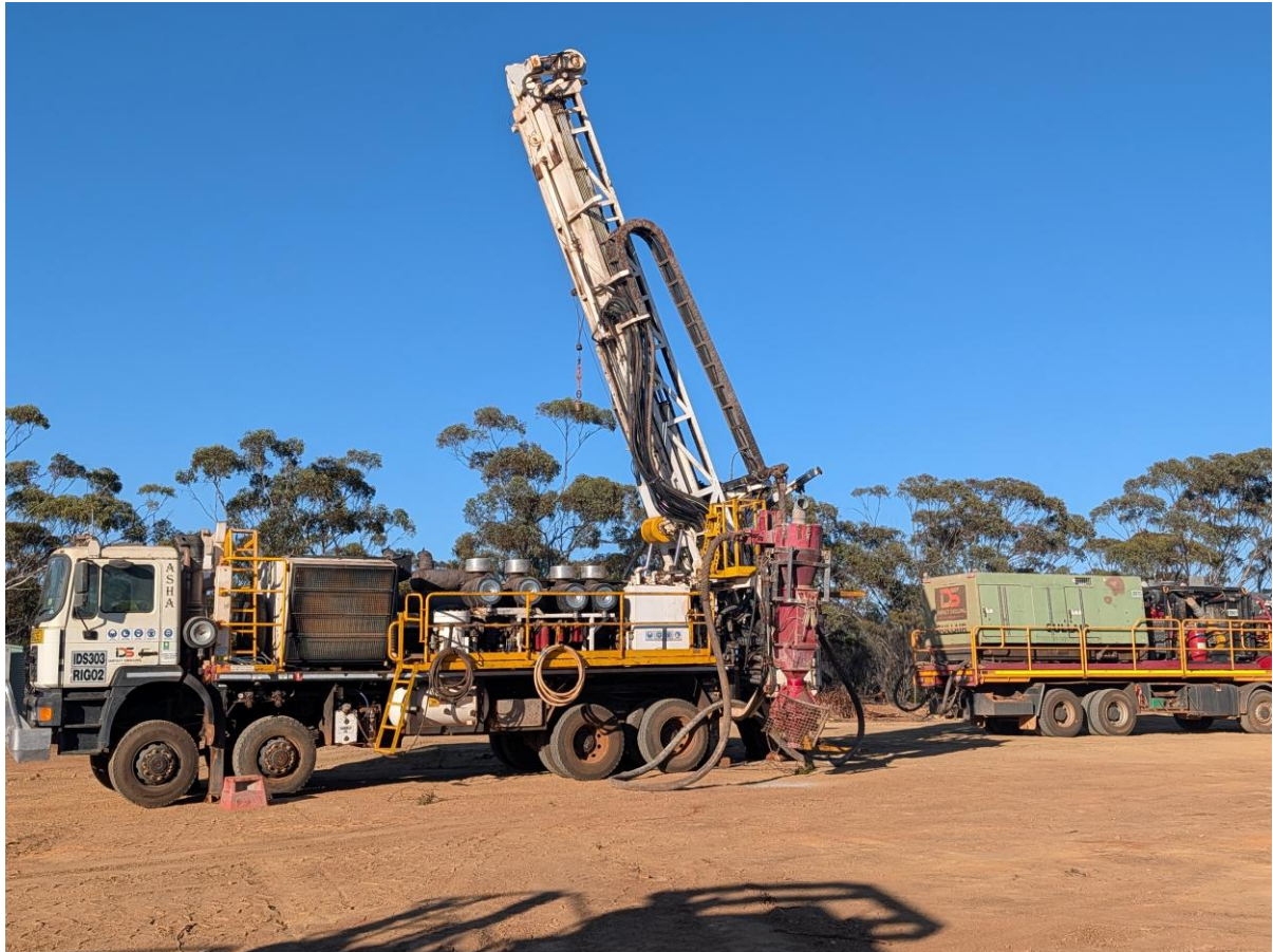
Figure 1 –Impact Drilling High Capacity RC Drill Rig Onsite At Van Uden
