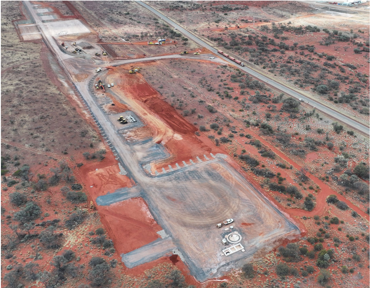
Figure 11: Earthworks and civils largely completed for the installation of 24 MW of wind turbines (4 x 6MW). Wind turbine components will be delivered to site commencing in November 2024.
