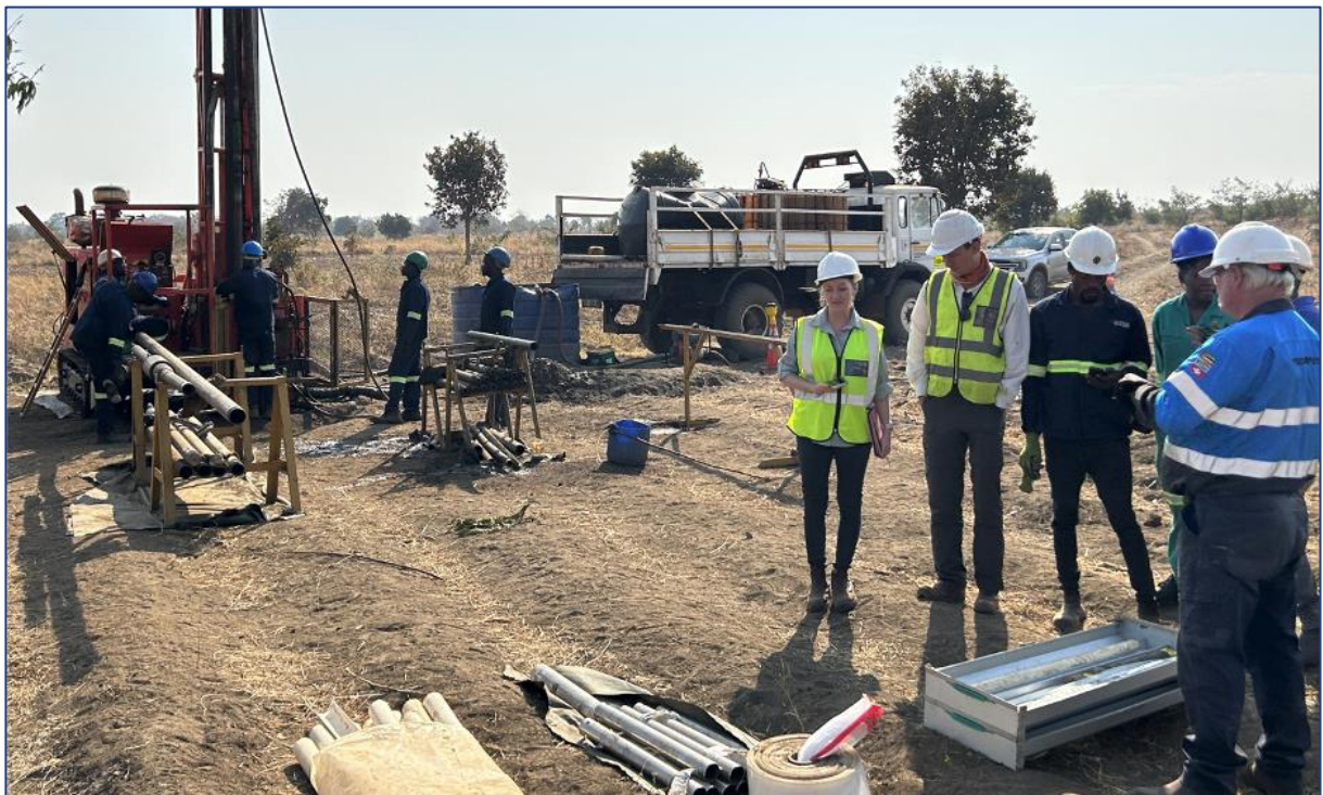
Figure 6: Push tube / diamond core showing stainless Shelby tubes for geotechnical samples and PVC casing for collection of push tube samples in foreground
