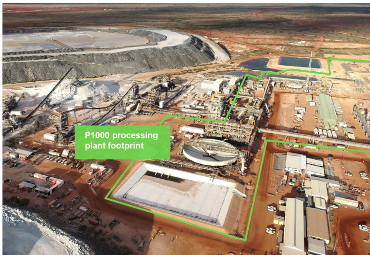
Figure 1: The P1000 Project as at 23 October 2024.
