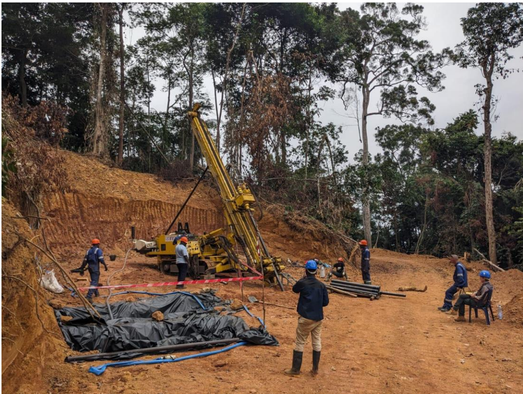
Figure 1: Rig drilling At P6.
