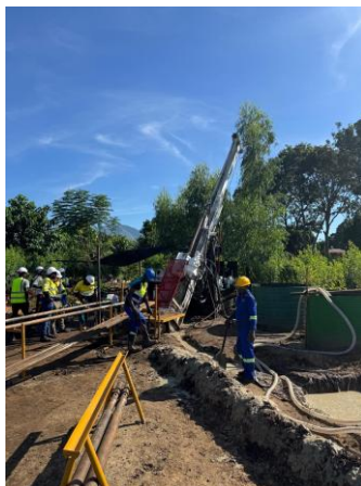
Figure 2 Diamond drill rig in operation
