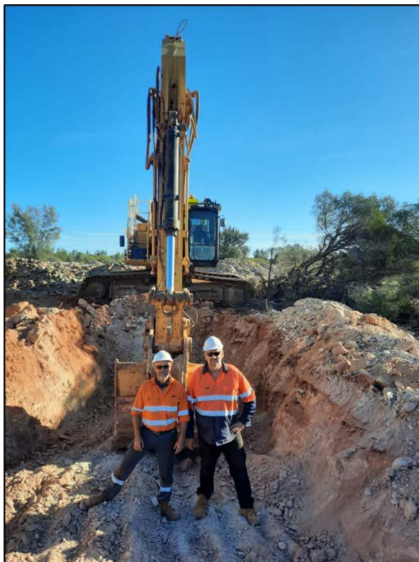
Figure 6: Contractor Lamington Minerals Pty Ltd crew onsite
