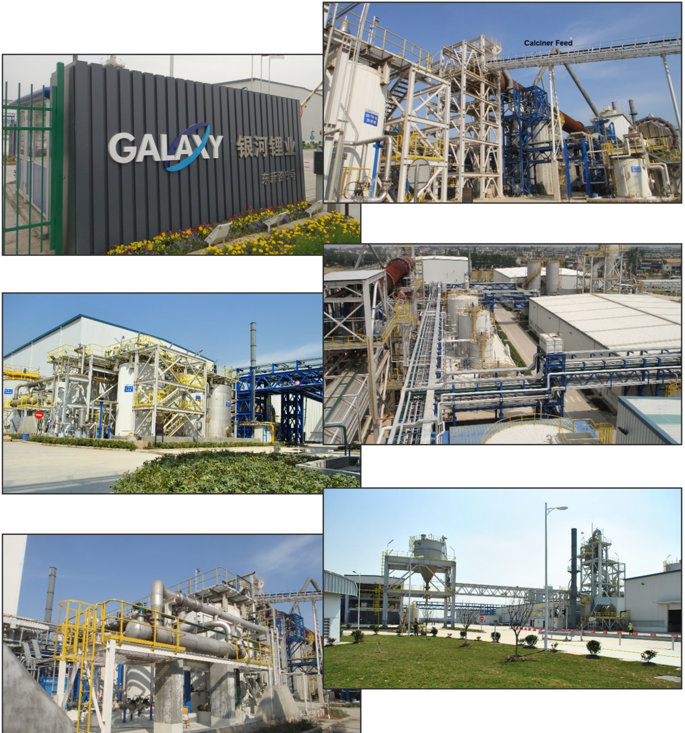
Figure 6: Galaxy Jiangsu Lithium Carbonate Plant
