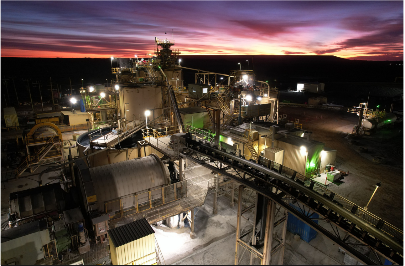
Figure 1: Lakewood processing facility is performing well.
