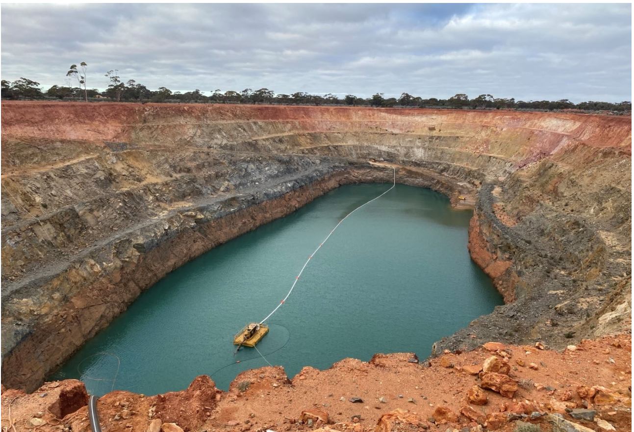
Figure 2: Dewatering infrastructure has been installed at Majestic ahead of portal development.
